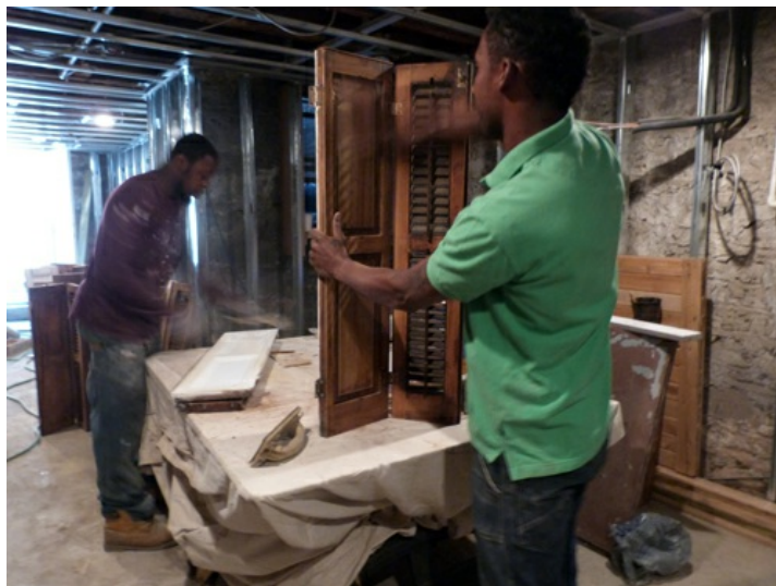
Workers restoring the original shutters
